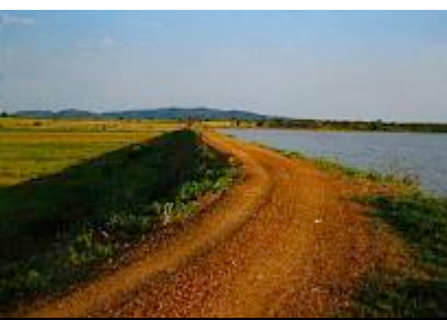
Earthen dam at Baraki
